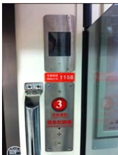
← using the VP-FD1 for installing with an intercom
